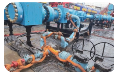
Fracturing project in Sichuan
