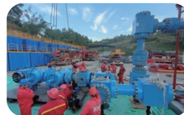
Fracturing project in Sichuan
