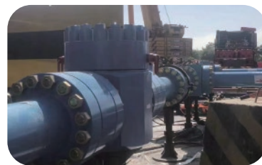
Fracturing Project in Sichuan
